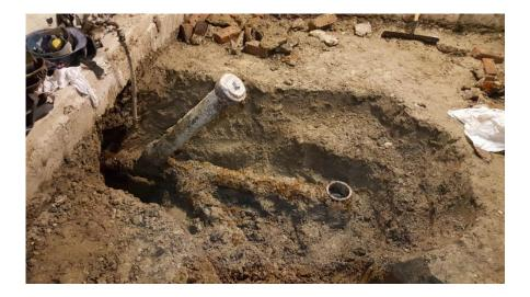
With the old gone and out of the way, the next step was to insulate and then pour the new floor. Note the thermal bridge between the old walls and foundation provided by rigid XP foam.
