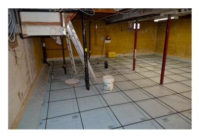
The new concrete floor was poured in place on top of 8 inches of XP foam, Poly vapour barrier, and new sewer lines plus weeping tile buried at the bottom. Note the new sump pit near the foot of the ladders. This completed the major work inside the house.
