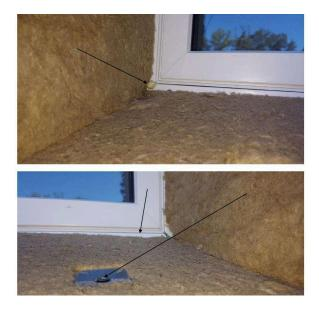
The doors had been fitted with fibreglass sills and the space between the new sill and the existing interior doors was temporarily filled with rigid insulation and rubber floor mat.
