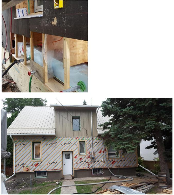
The Larsen Truss cavities were then filled with dense-pack cellulose. Areas under the windows were filled first through access holes that were later sealed (see red tape in the
