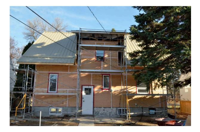
With this weather barrier in place, work could proceed on the exterior of the foundation walls. This included blueskin on the sealed surface of the concrete walls and the top of the exposed footing. The weeping tile around the footing was replaced along with clean drainage rock.
